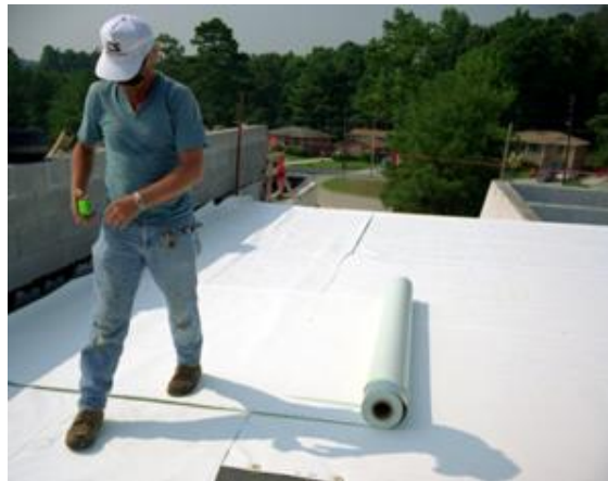
Figure 1: Installation of a ‘white roof’ 72
